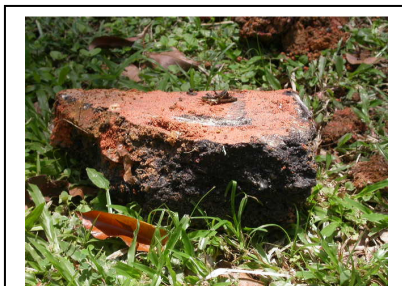
Trace of broken tarmac found in this trial pit
